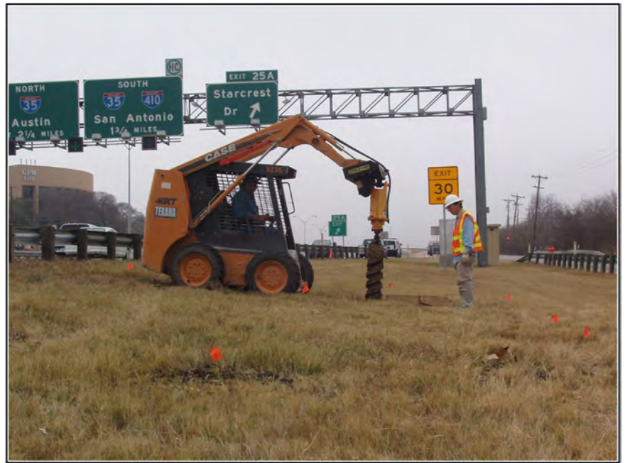
Figure 4-17. Auger testing in the median at the Granberg Site.
